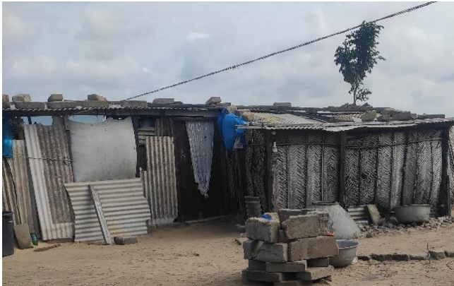
Figure 5: Makeshift shelter constructed with coconut leaves and salvaged materials. Source: Own photo with the permission of the residents.
